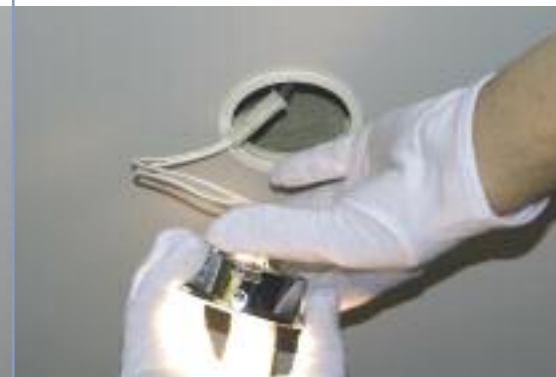
Downlight einbauen Installing the lighting
