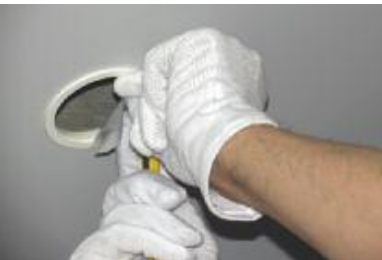
Decke innen im Ring wegschneiden Cutting away the vinyl on the inside of the ring
